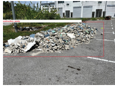
CONSTRUCTION WASTE Debris and unsecured site spill
