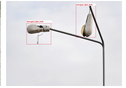
BROKEN LAMP POST Damaged lighting & utilities
